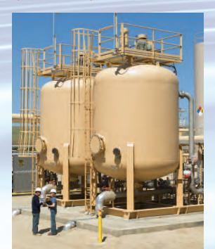
The success of the Power Clean® media cleaning process is the fluidization process that easily strips contaminants and oil from the media, using very low volumes of backwash water without the use of surfactants or gas/air scour.
